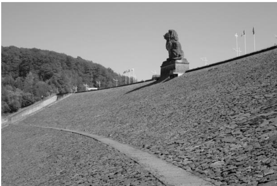
The dam at La Gileppe.
